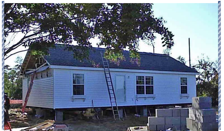
Cottage 6 on its foundation and roof up!
