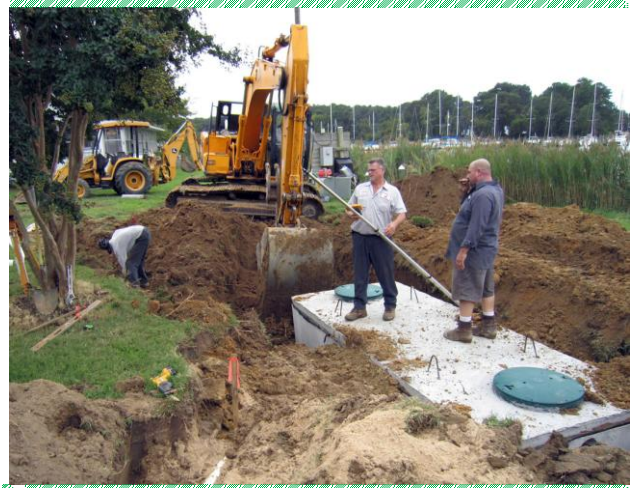
Installing the Septic Tanks next to the Houchen Cottage
