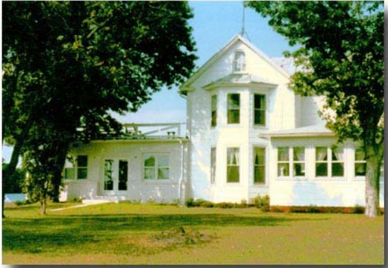
Re-located doors to side of Bean Room
