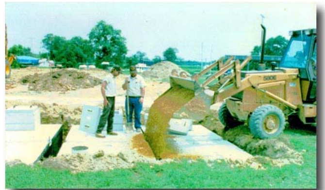
Right: Septic System Upgrade
