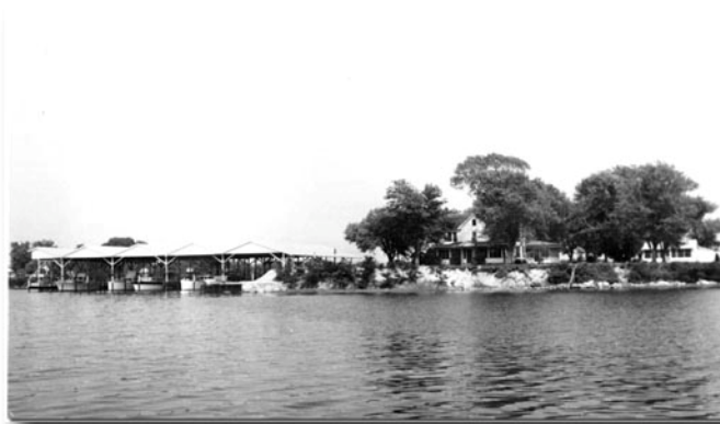
CYC taking shape with construction of A-Dock sheds
