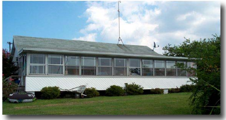
Original "Clubhouse" then "Kid's Clubhouse now "Cottage 2"
